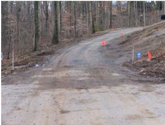
Drive Entrance Before
