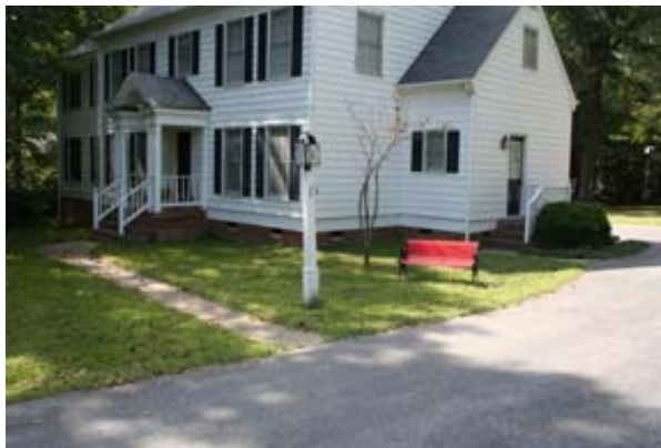
Front Door Entrance Before
